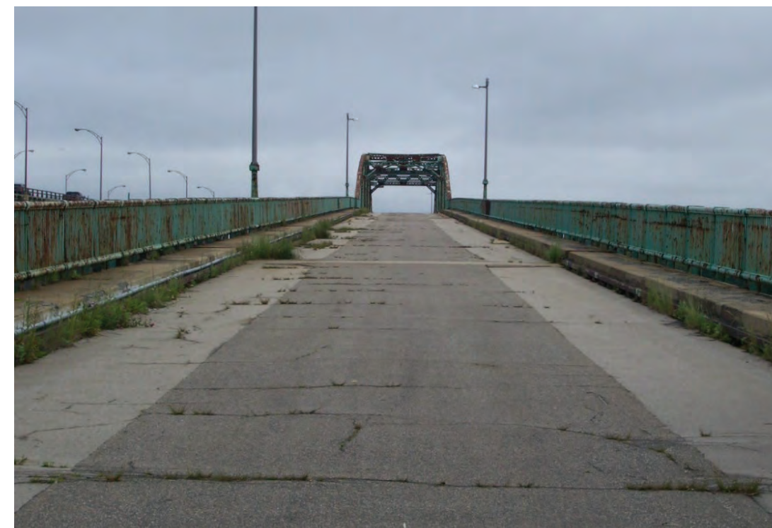
4. Pedestrian view south on GSB deck without fencing, facing Newington. June 24, 2009.
