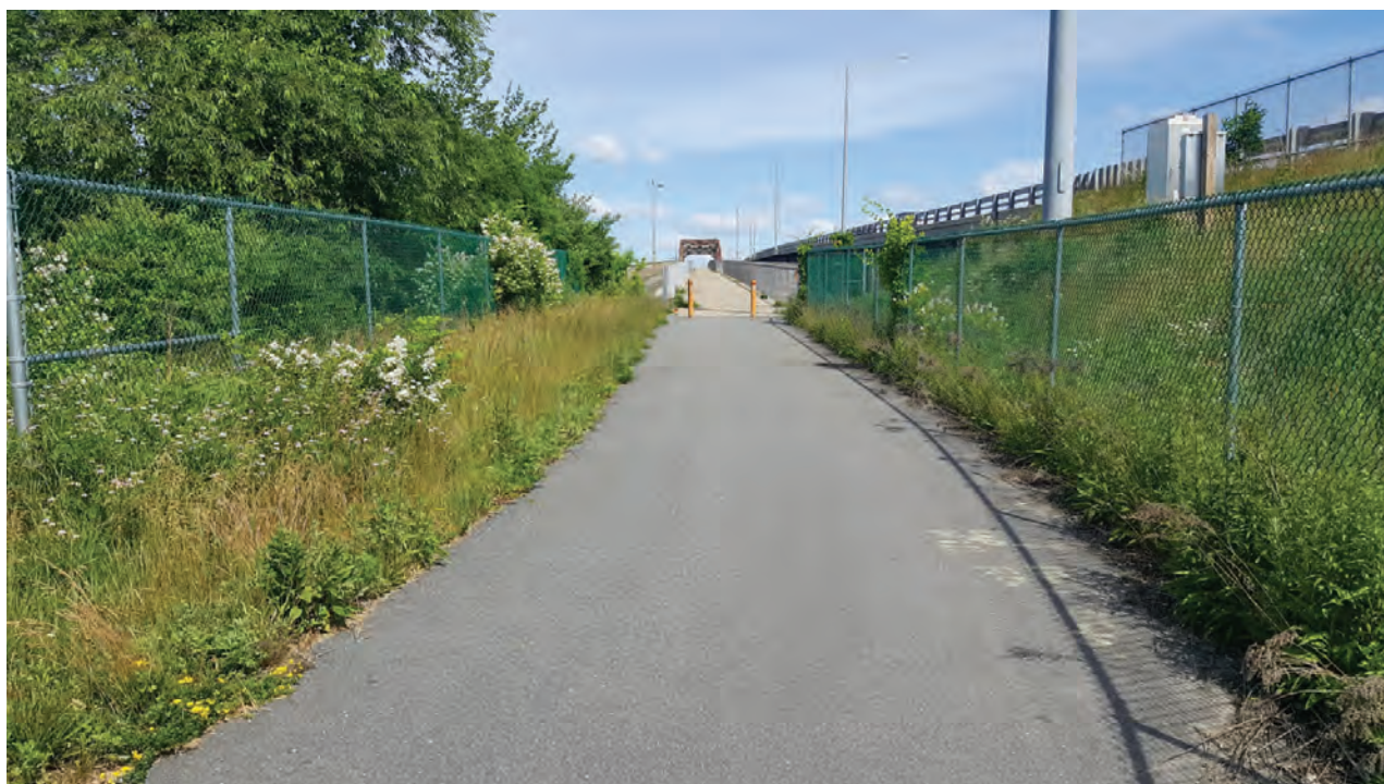
2. Newington side – pedestrian view north toward the GSB from the approach. June 19, 2018.
