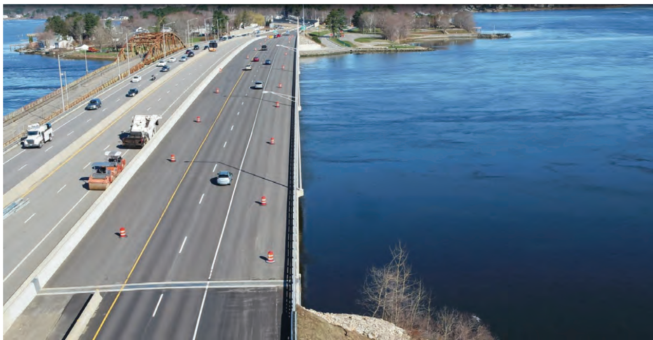
1. Aerial of the GSB and LBB decks over Little Bay, view north (toward Dover). April 17, 2019.
